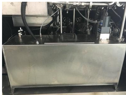
Pipe and valve
